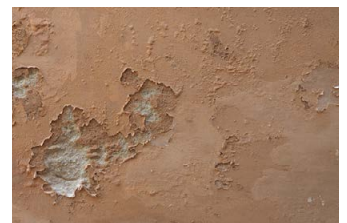
Damage to wall caused by flooding.
