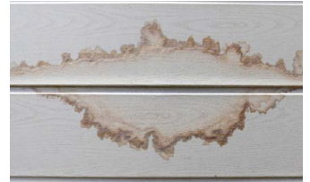
Water stained ceiling panels.
